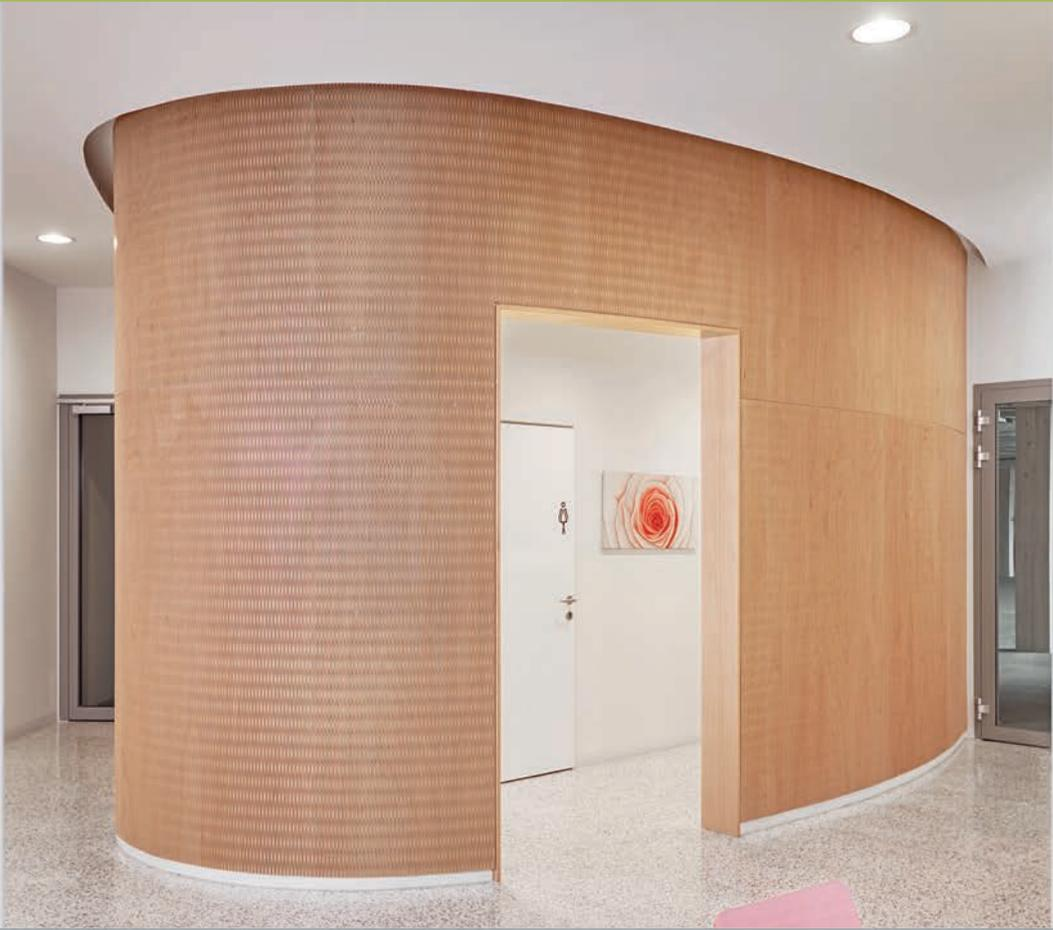
dukta® LINAR in Multiply beech with white fleece backing used to clad the curved wall surfaces in an office building.
